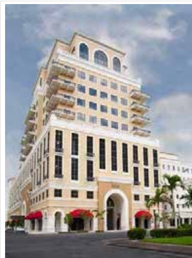
2020 Ponce contains a total of 130,000 square feet, including ground-level retail, seven stories of premium office space, and a six-level parking garage.
